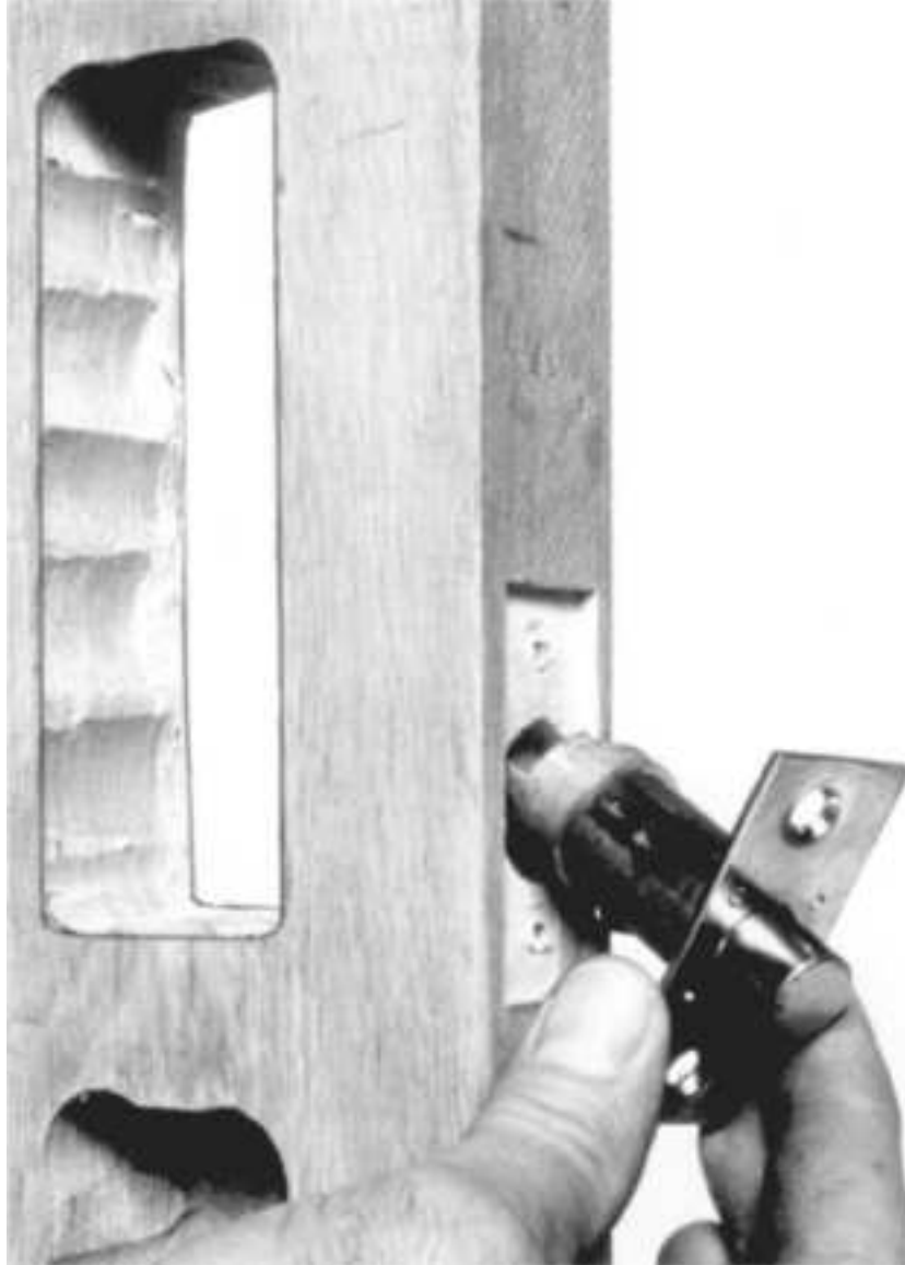
Figure 18.49 Preso-Matic installation, Step 3.
